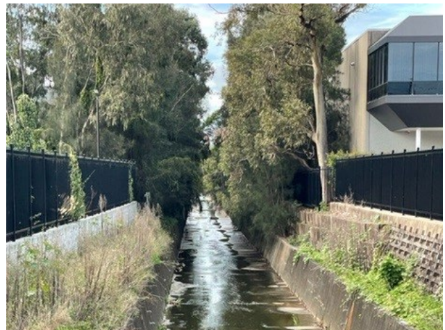
Picture 8 Haslams Creek to the west
