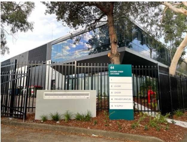
Picture 7 Warehouse to the south
