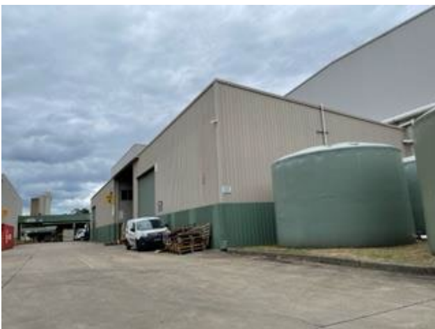
Picture 1 Loading docks & water tanks
