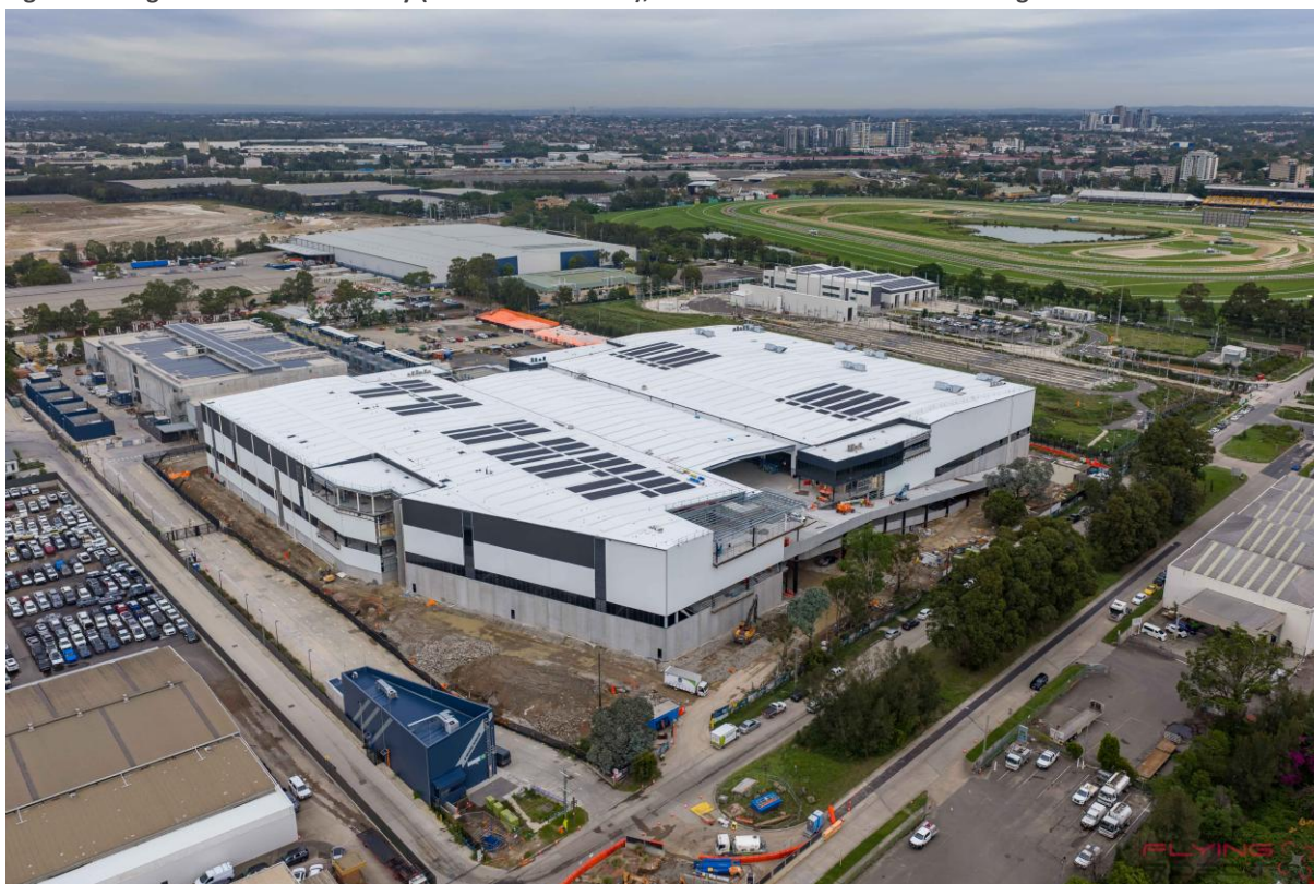
Figure 2: Image of the site and facility (under construction), view across Grand Avenue looking southwest
